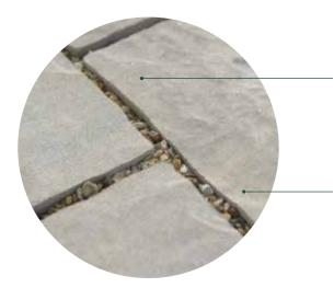
The pavers used in a permeable installation look similar to traditional pavers, but are made with special spacer bars that create a wider joint.
